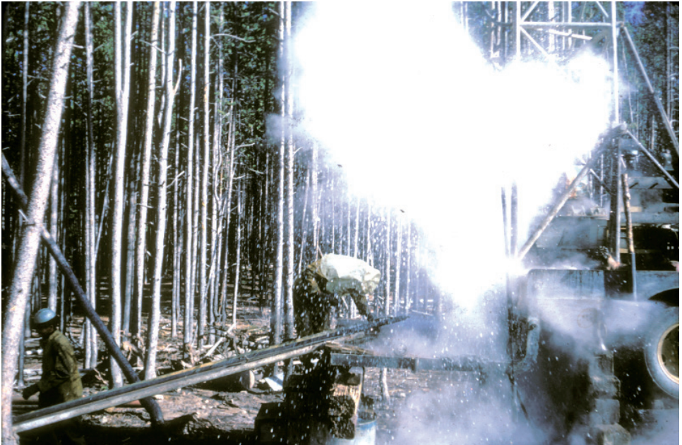
Photograph of eruption of steam from the drill rods in drill hole Y-9, Norris Geyser Basin, Yellowstone National Park, 1966. The driller and his helper (with white hood) are moving rapidly to escape the steam exploding from the drill rods.
